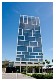
Figura 1.9: Port Corporate Tower
